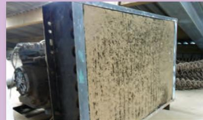
Poor ventilation means that it is difficult to get hot air away from the condensers which causes their efficiency to fall. Ideally, coils should be located in an area with good ventilation and away from direct sunlight – preferably North facing. If the area around the compressor set is being used to dry clothes it can show that the condenser isn't getting rid of the heat effectively, thus lowering the efficiency.
