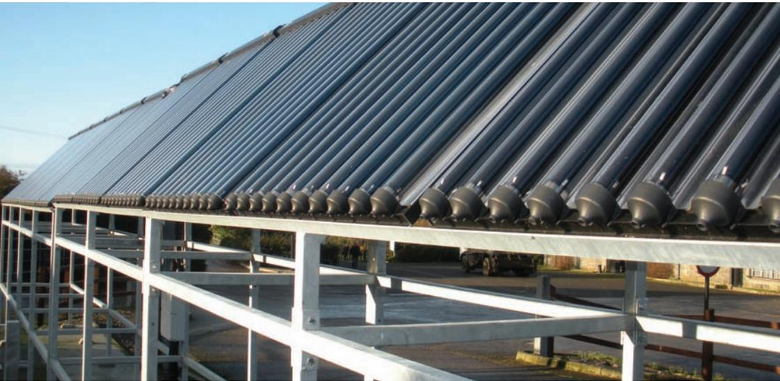
Evacuated solar heat tubes give the best thermal performance. As well as working well in bright summer conditions, they have the potential to provide some heat even in colder overcast and winter conditions.
