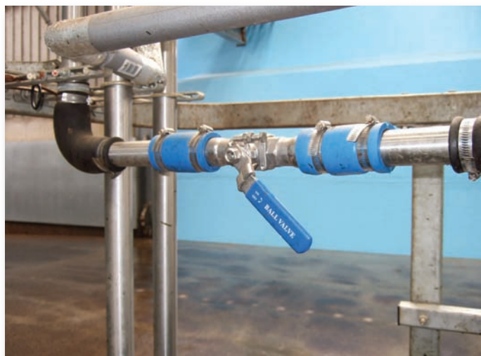
Partially closed ball valve
