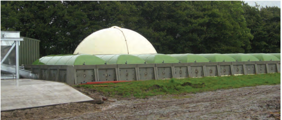
An example of a small scale AD plant
